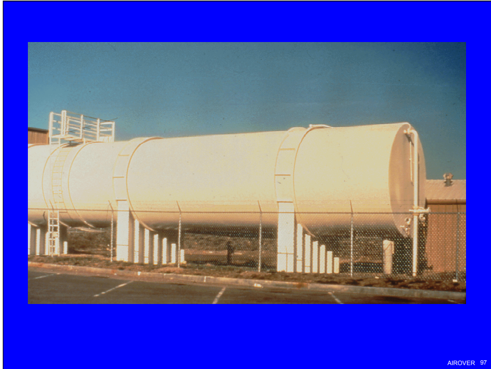
40,000 gallon horizontal tank. Note manway at top, fill or overflow piping at end, and sonic level measure at top above far right support.
